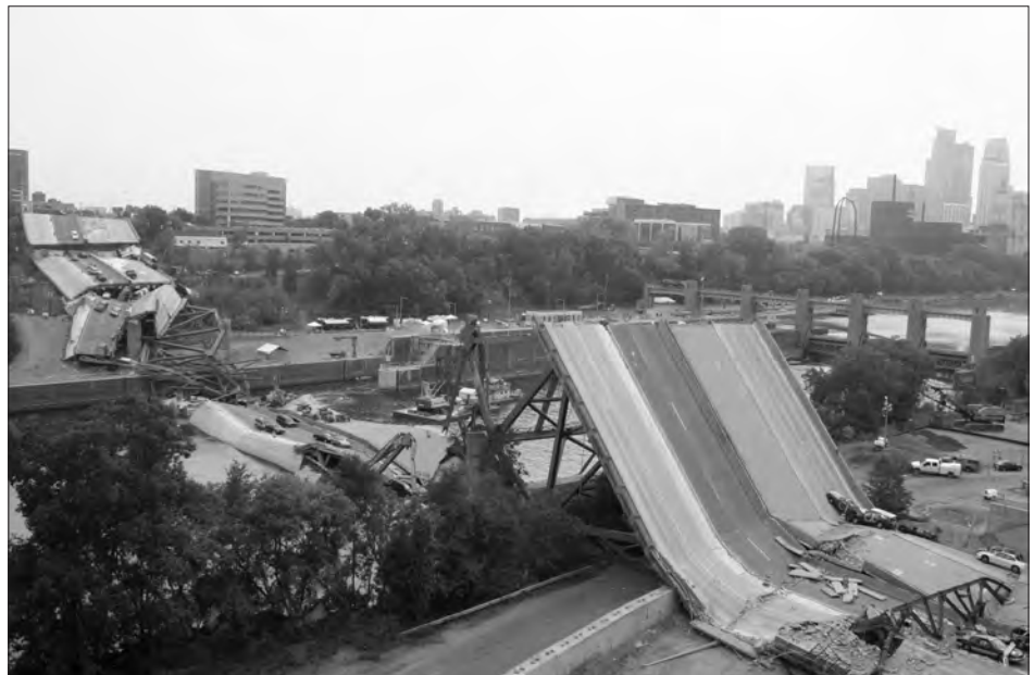
The collapsed I-35 bridge over the Mississippi River in Minneapolis, MN. (Photo: Courtesy of the Hennepin County Public Affairs Department)
